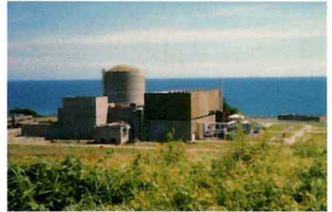
This nuclear power plant has been mothballed using 15 Munters dehumidifiers—a very cost-effective, long-term solution.
